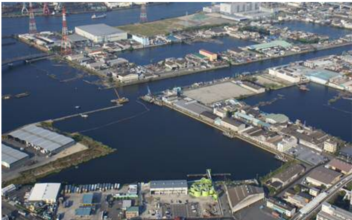
Figure 2. No.6 Lumber Yard (before the project)
